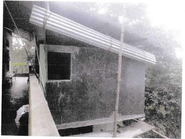
Rain Water Harvesting
